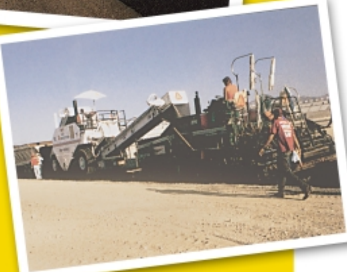
Las Vegas Paving lays the first layer of the asphalt concrete pavement leveling course on turn 3 of the Las Vegas Motor Speedway tri-oval.
