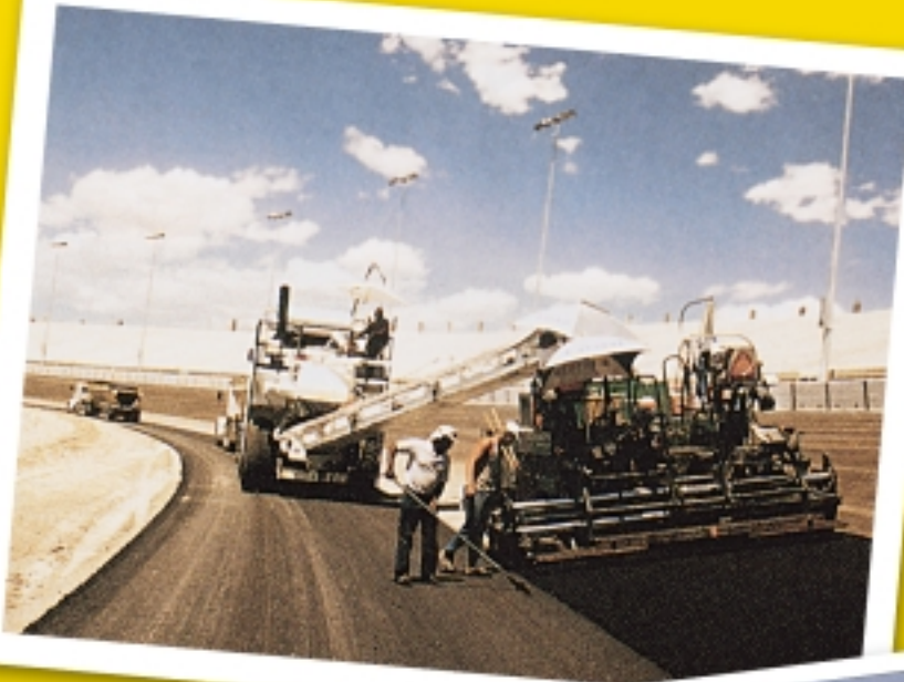
A Las Vegas Paving crew places the racing surface on the road course at the Las Vegas Motor Speedway.
