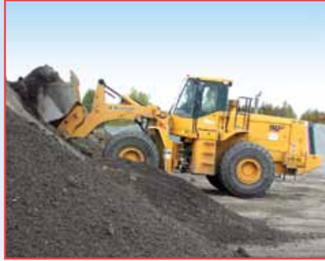
K.J. Beamish Construction Co. operates its own pits and quarries.
